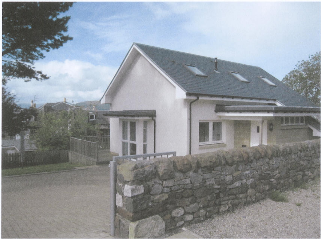
Building 11 - Window Type: UPVC Various Openings
