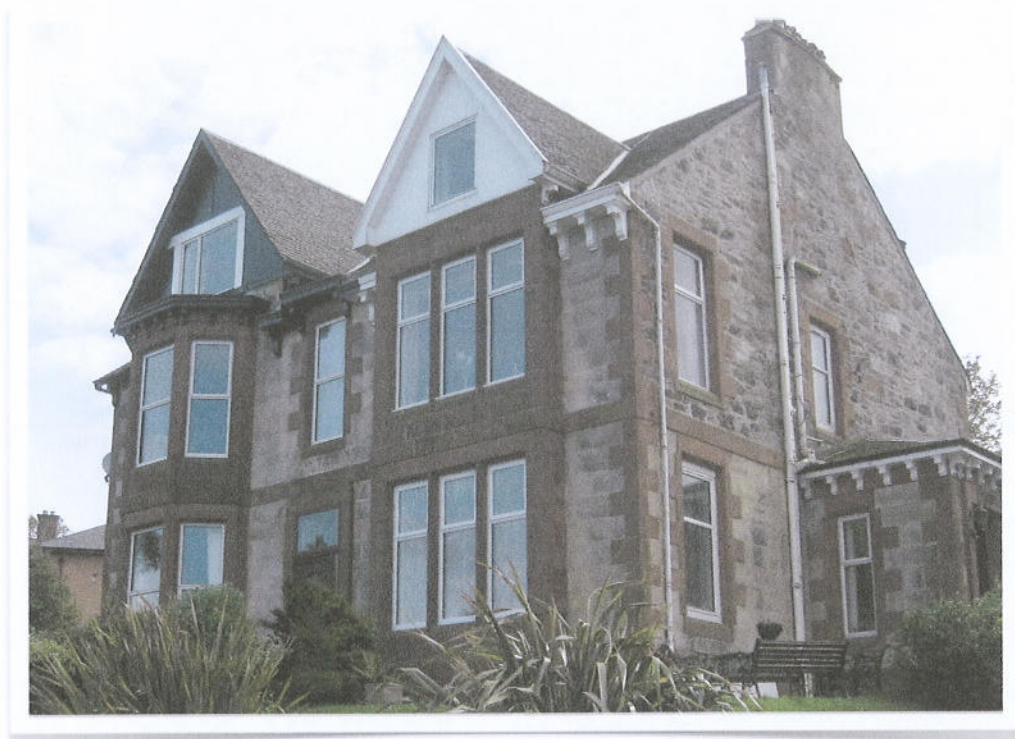
Building 32 - Window Type: UPVC and Various Openings
