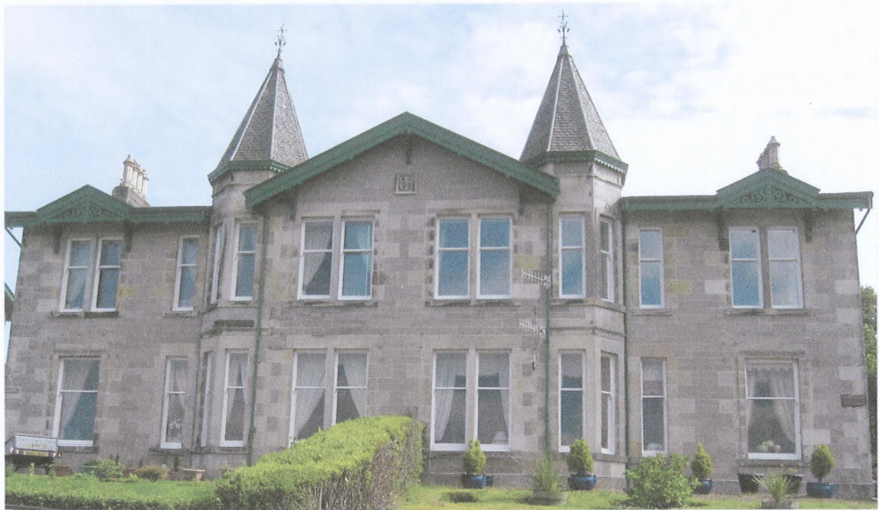
Building 16 - Window Type: Original Installation
