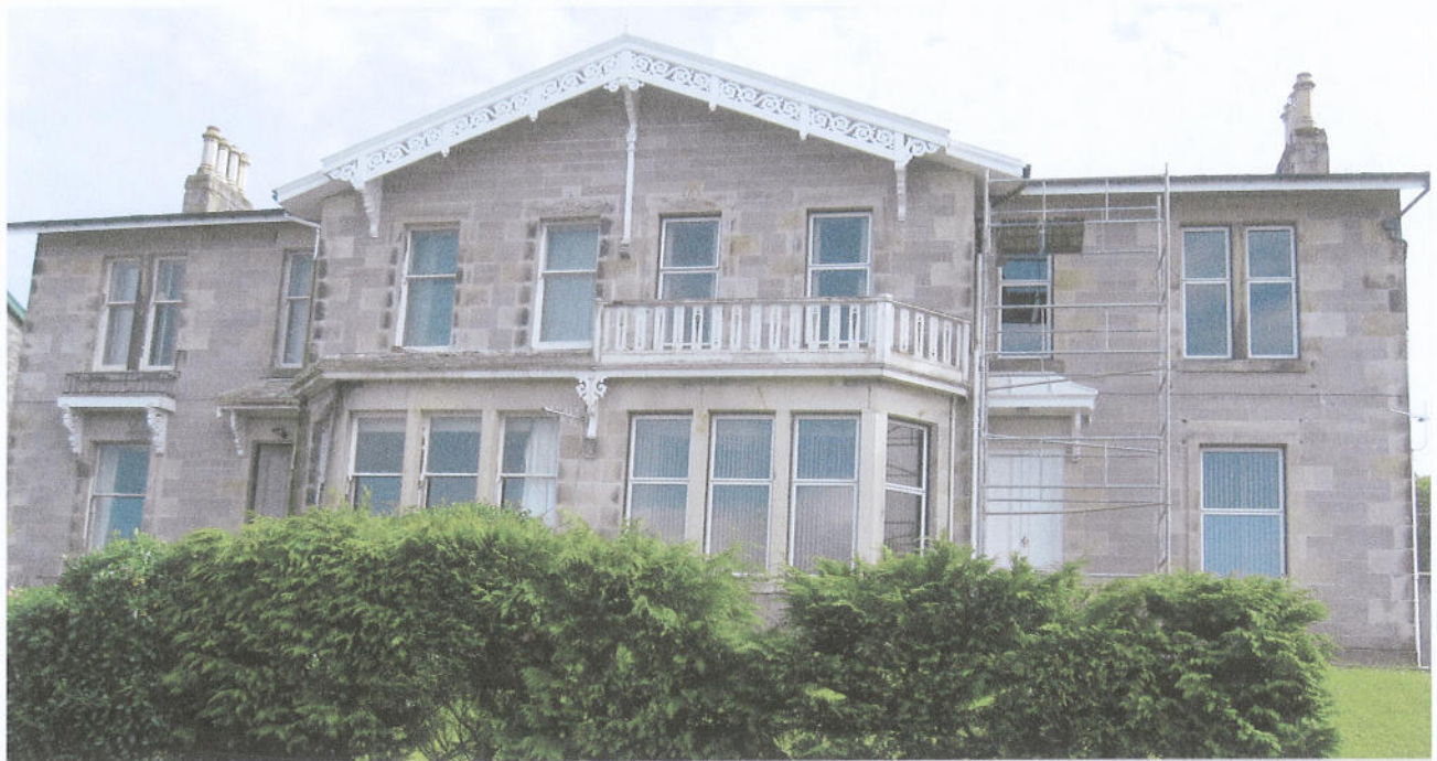
Building 15 - Window Type: Aluminum, Original Installation and Various Openings
