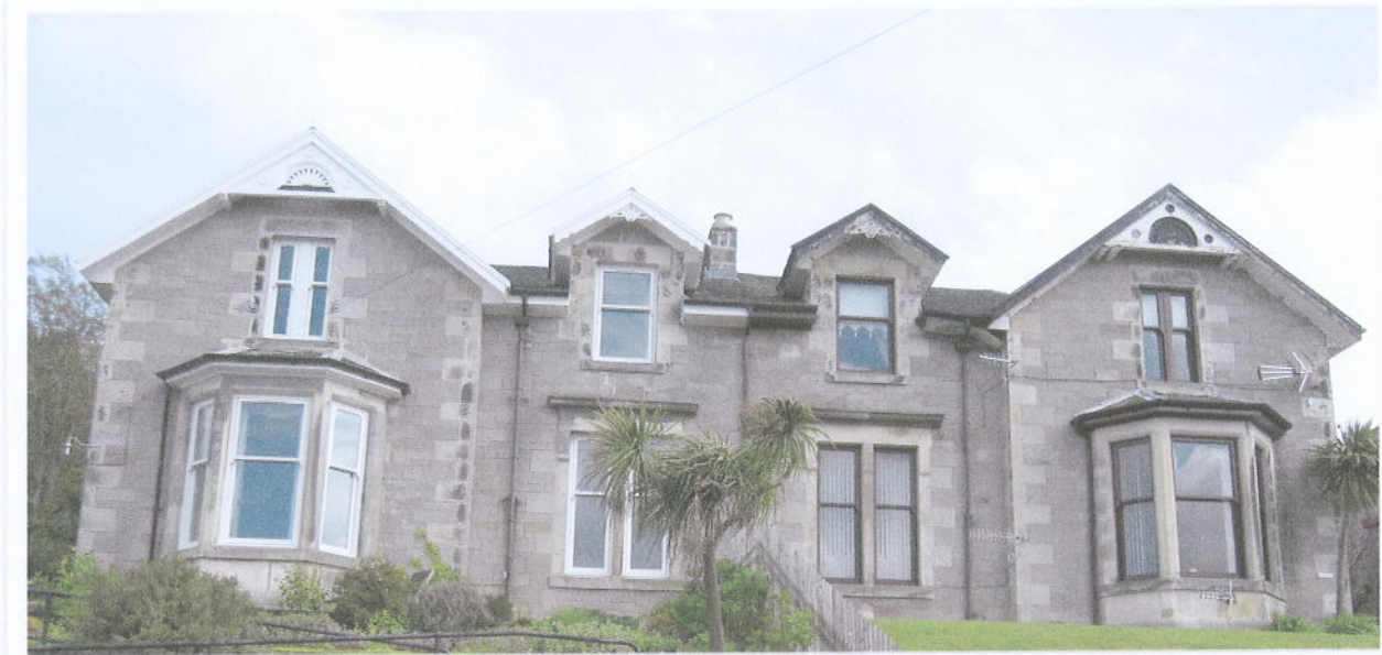
Building 3 - Window Type: Wood Double Swing & Various Openings
