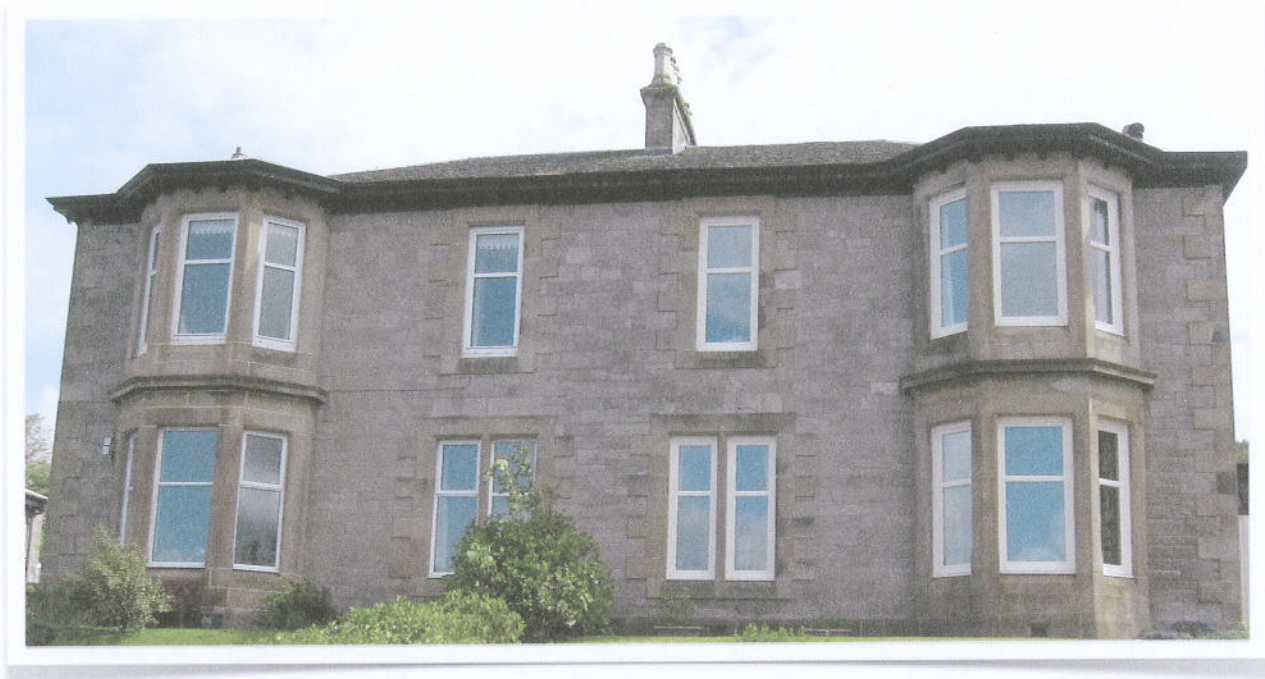
Building 30 - Window Type: Aluminium, UPVC and Various Openings
