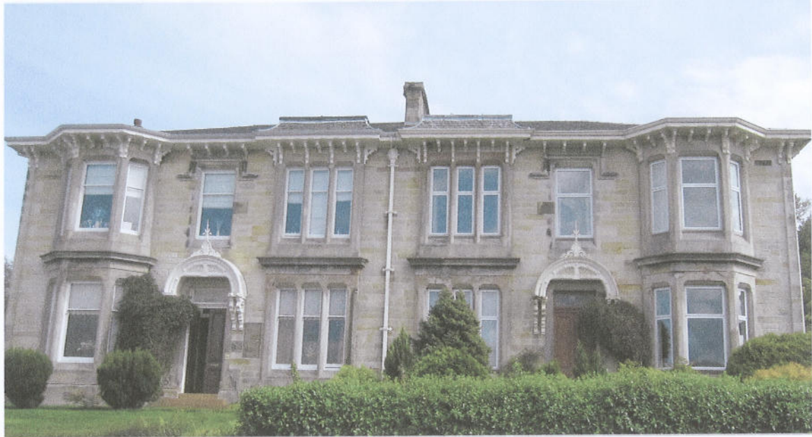
Building 7 - Window Type: UPVC, Aluminium, Original Installation Various Openings
