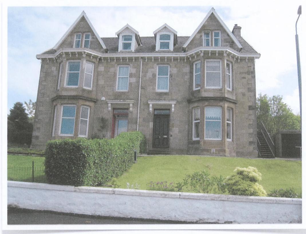
Building 26 - Window Type: Original Installation
