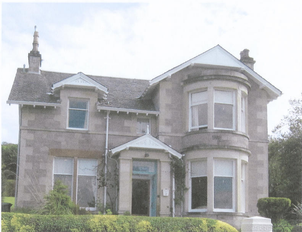
Building 12 - Window Type: Original Installation
