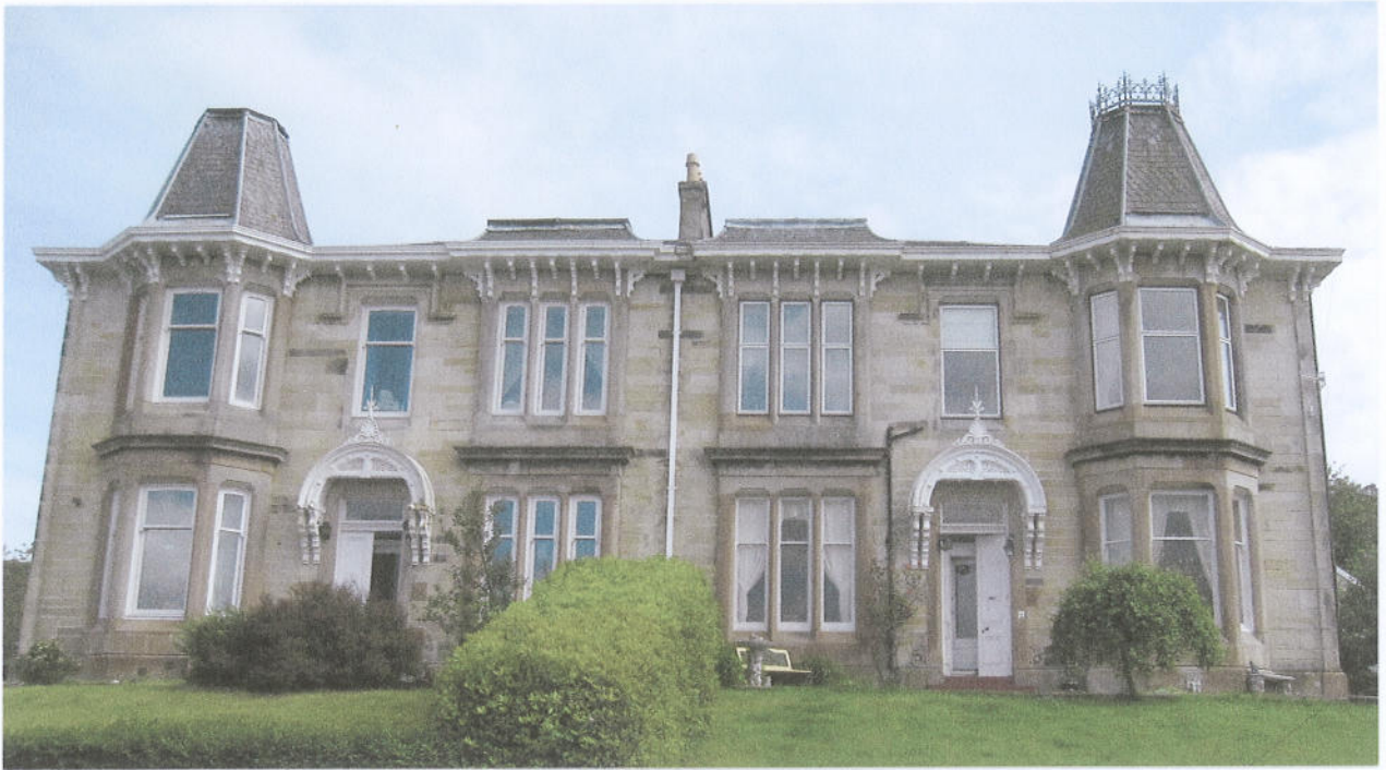
Building 9 - Window Type: Wood Double Swing, Aluminium, Original Installation and Various Openings
