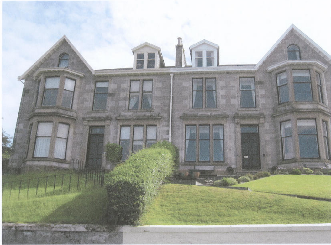
Building 23 - Window Type: Original Installation
